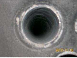
The tubes are in excellent condition, very light scale in places. Minimum reduction in Heat transfer rates
