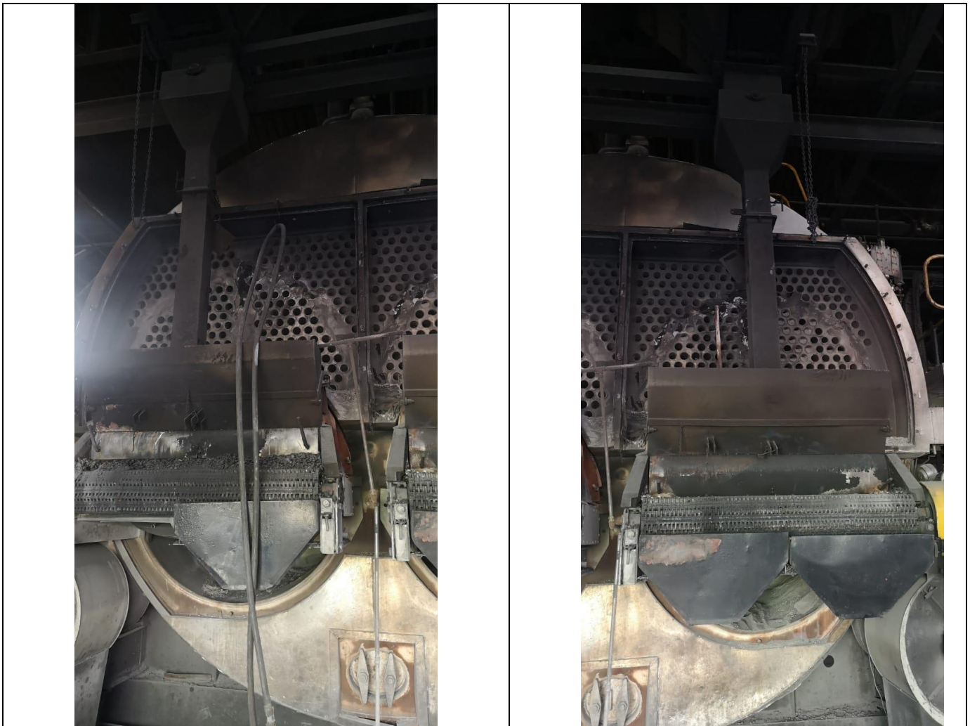
Frontal of Left and right smoke boxes. Opened prior to cleaning
