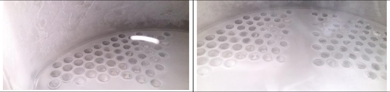
Right Hand Reversal chamber clear after 1 year operation
