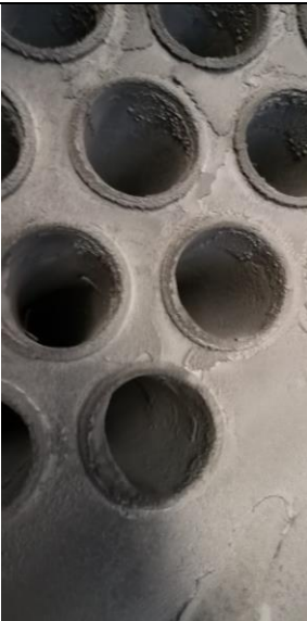
Ash build-up of more complete combustion
