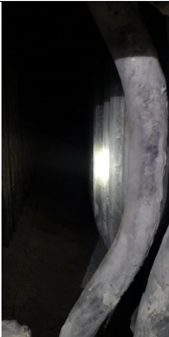
Superheater entry no 2, paper thin deposition removes with a plank
