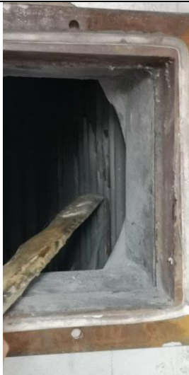
Superheater entry no 2, paper thin deposition removes with a plank
